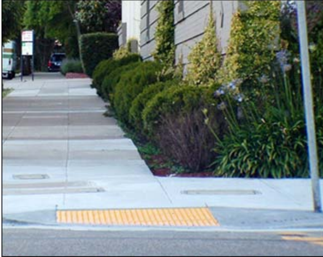
Figure 28. The intersection of the outside sidewalk edges is the right-of-way corner.
